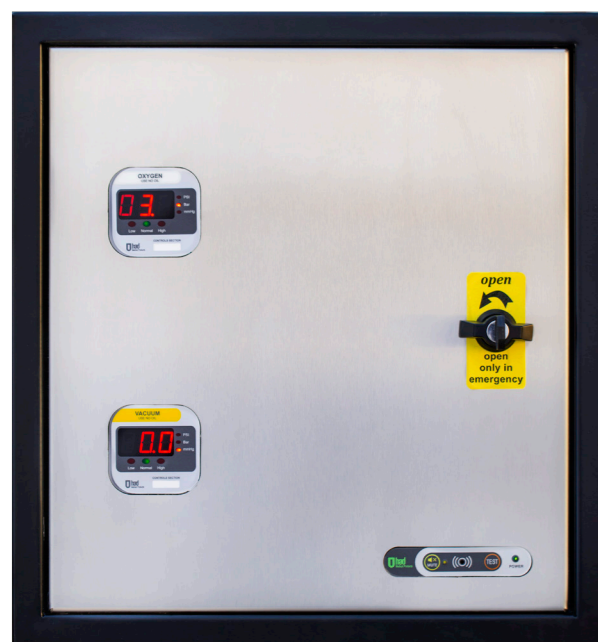
Control Valves Medical Gas Systems
